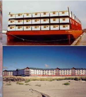
Prefabricated Structures (Precast or Modular)
